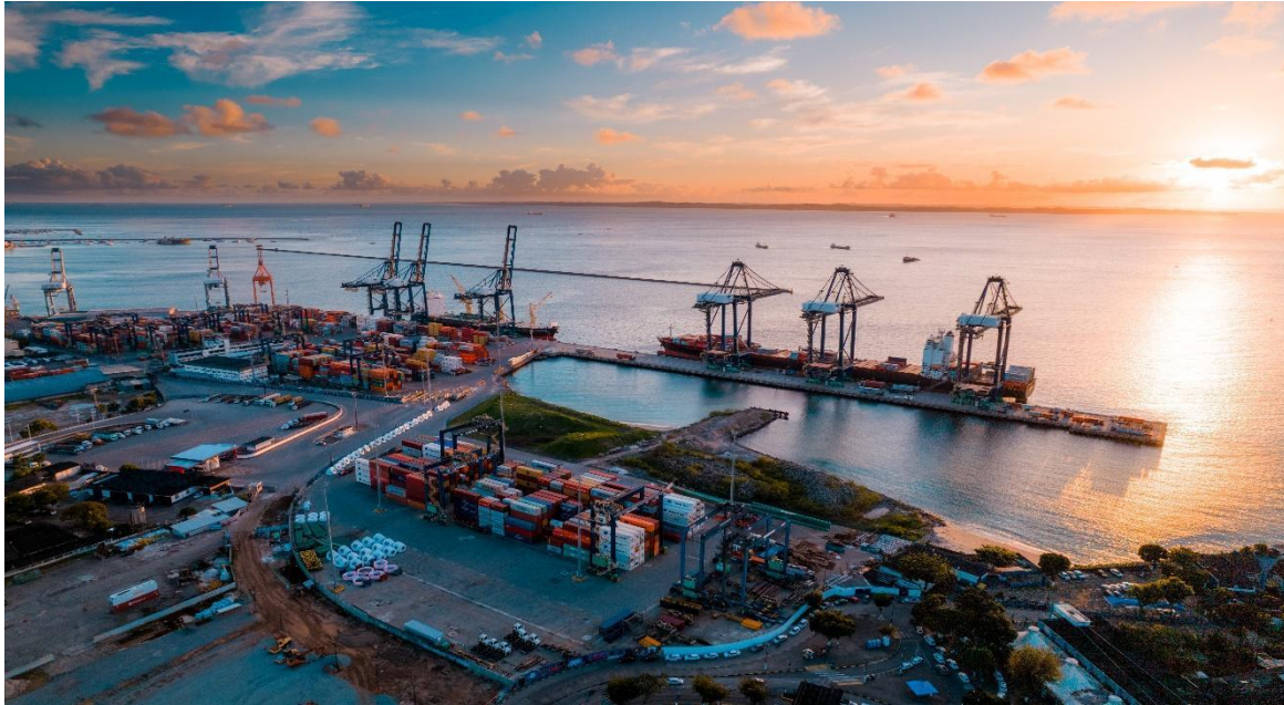
Wilson Sons: Salvador Container Terminal can receive 366-m ships with cutting-edge equipment
